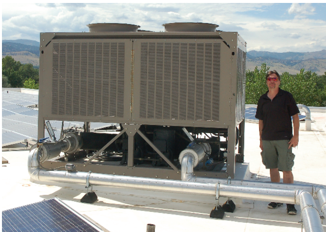
Figure 1: 40-ton air-cooled chiller. Air-cooled chillers use fans to reject heat by drawing air across the condenser.
